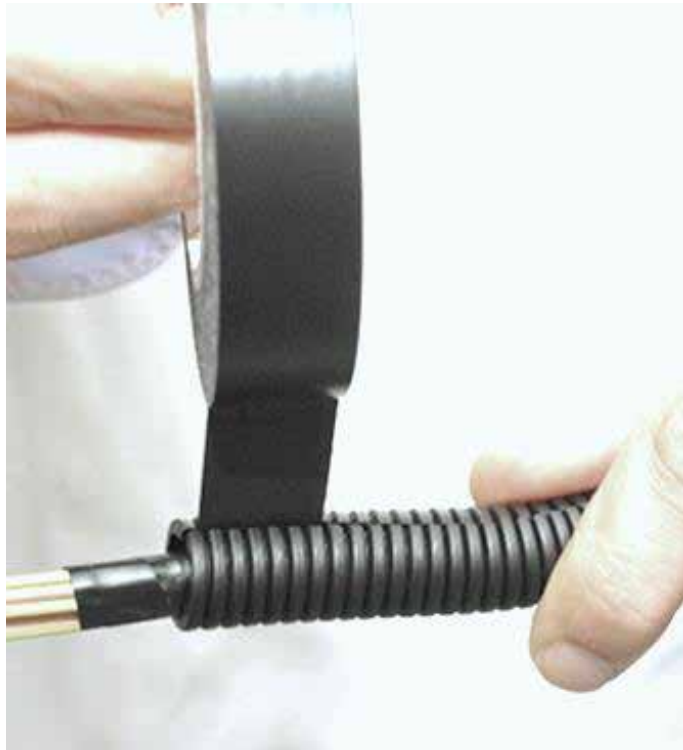
Start to fix the tape on the harness.
