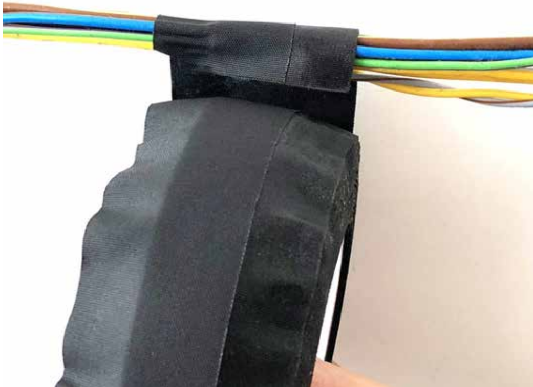
Fix the tape on the harness from the rear
