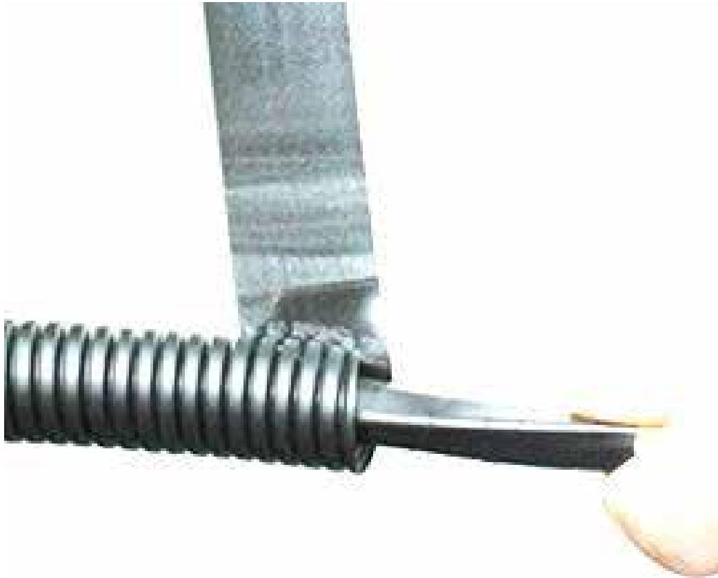
Additional triple winding on the corrugated tube
